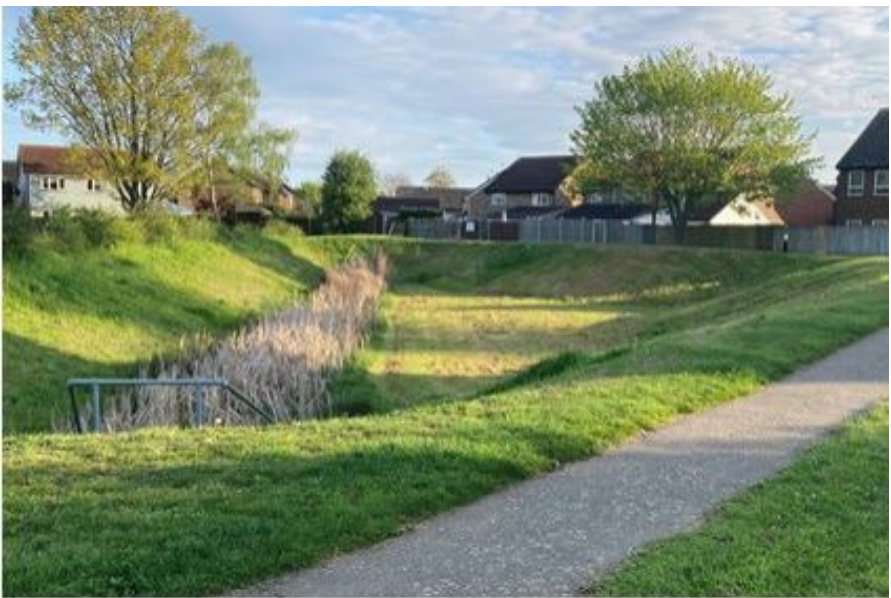
^ example of SuDS attenuation basin as part of sitewide drainage strategy
