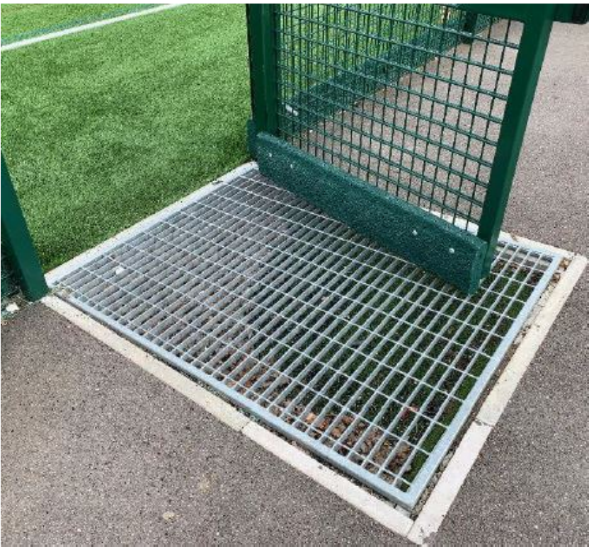
^ example of detox grids and low-level trek boards to manage rubber crumb
