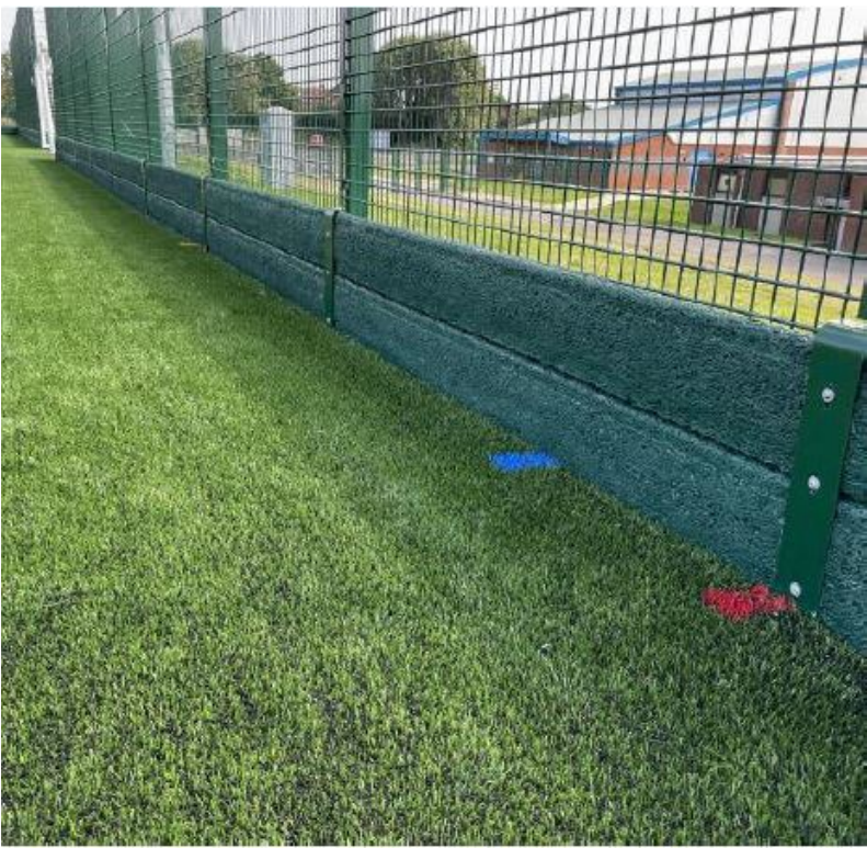
^ example of detox grids and low-level trek boards to manage rubber crumb
