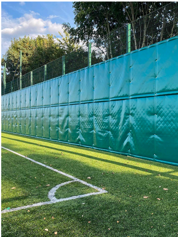
^ examples of acoustic quilting and fencing with ballstop fencing
